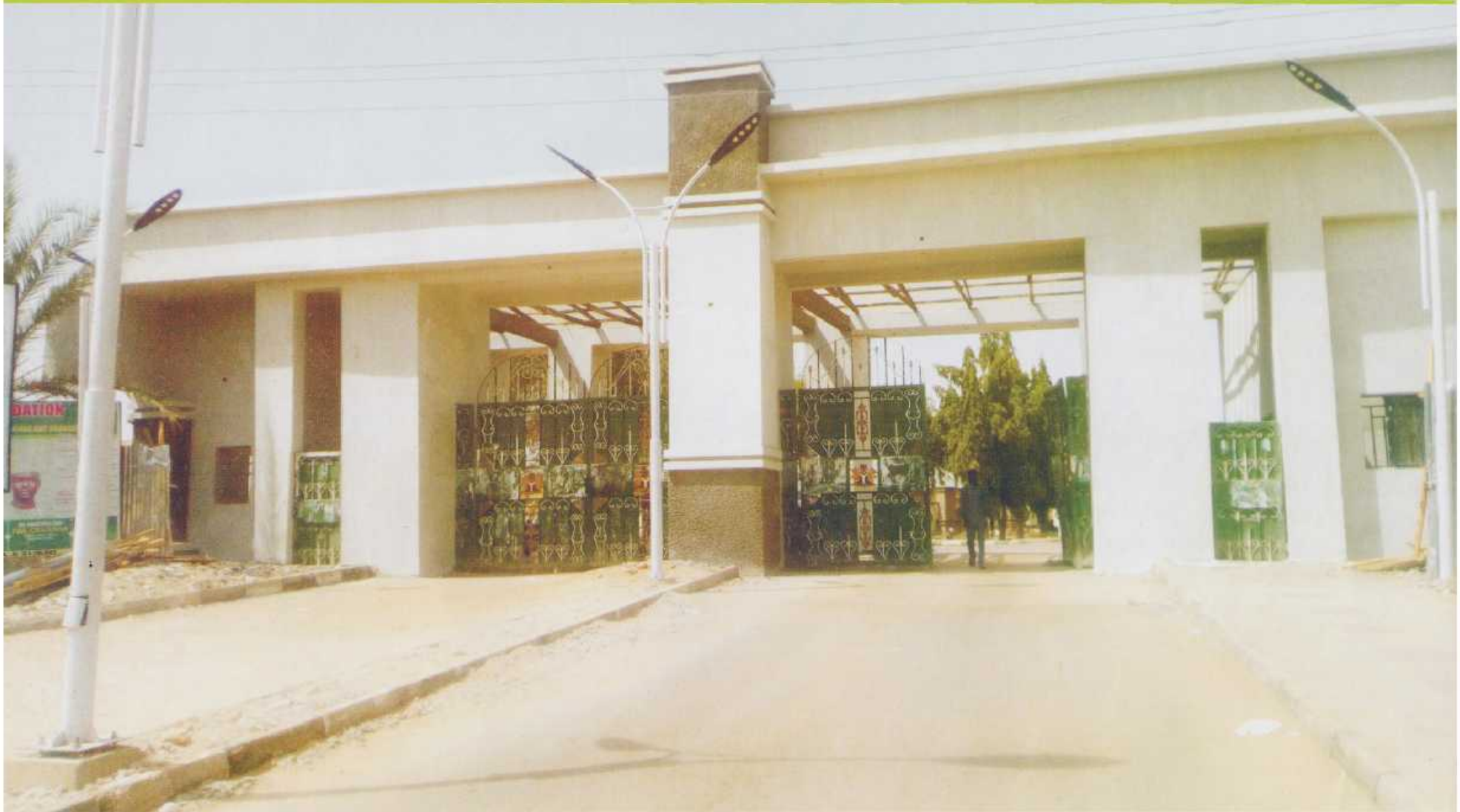
The Newly Renovated Zamfara State Government House, Gusau
